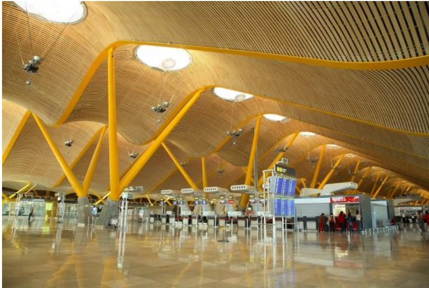
Figure 17: Bamboo is increasingly adopted by Western architects as building material, for example the Barajas international airport in Madrid by Richard Rogers (Photo MOSO International).
